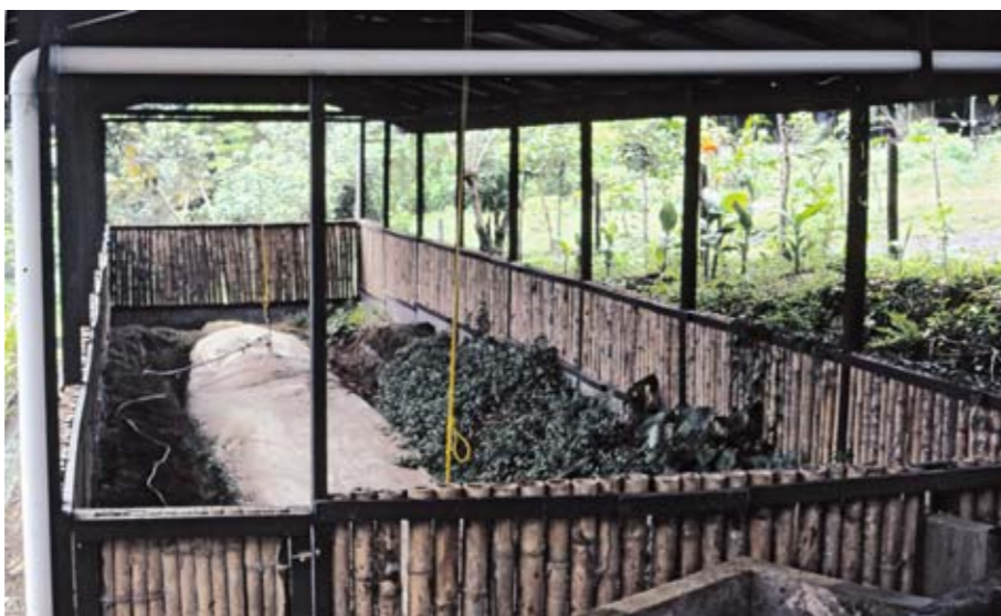
One of the points of interest is this biogas plant made to help heat the water.
