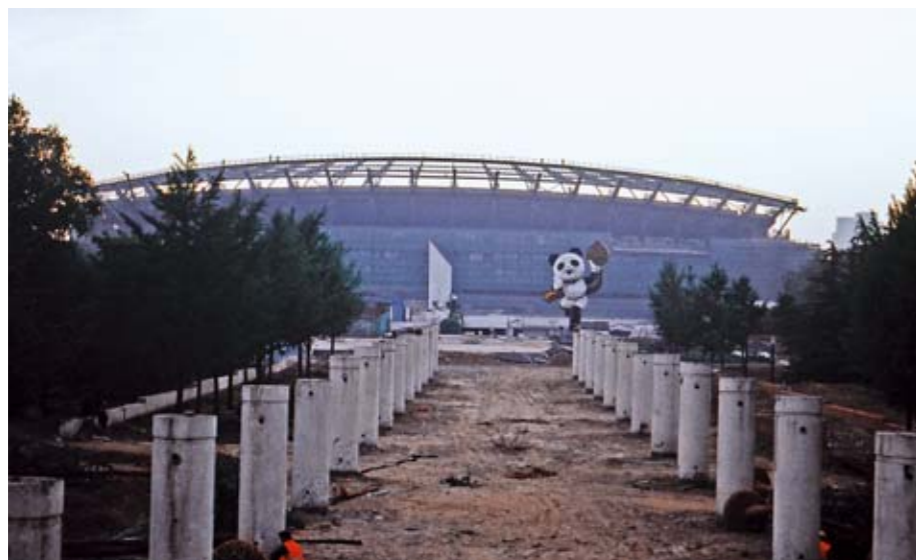
Another Olympic stadium, in 2007 still under construction.
