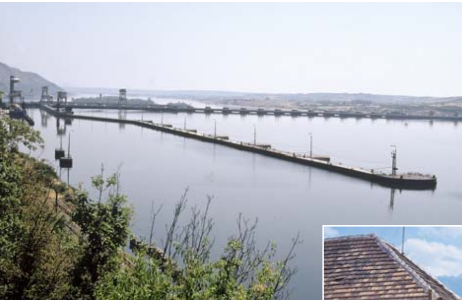
The large water project Iron Gate, which was built between 1946 and 1972, is quite close. The dam is 1,200 meters (3,940 ft) long and 63 meters (207 ft) high. After completion the dam raised the water level of the Danube by 33 meters (108 ft). The hydroelectric power plant has an output of 2,100 MW (equivalent to two large nuclear reactors). The electricity generated goes into the two countries.
